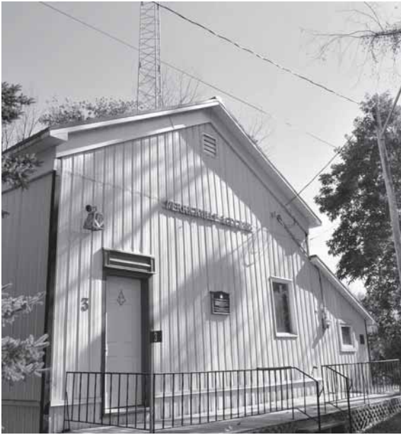
Sponsored by Merrickville No. 55, a communication tower rises up above the Lodge Building in Burritt's Rapids. Dedication took place on Sept. 11, 2010.
